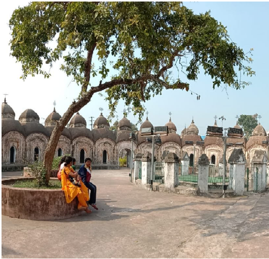
Fig. 2 Tree provides shade Kalna, Burdwan, W.B.
